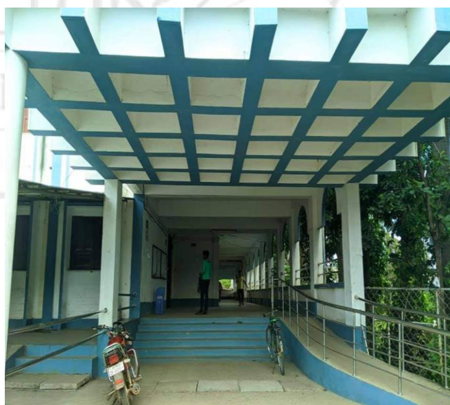
Ground Floor Entrance
